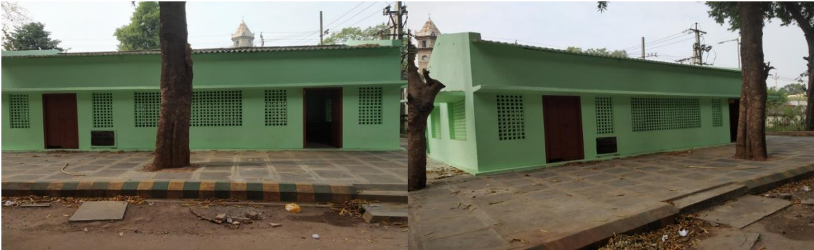
Construction of Toilets
