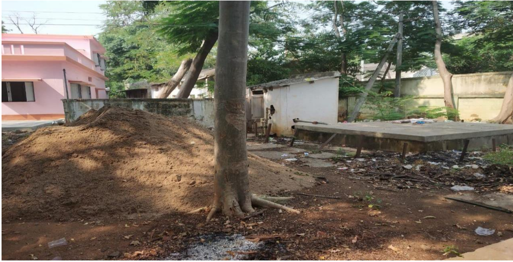
Waiting hall Renovation
